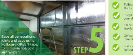
Foilboard® Panels don't need to join on a batten or purlin. Butt join and tape to ensure continuous insulation.
